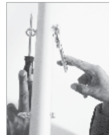
Figure 9: Use two fingers to tighten bolts
